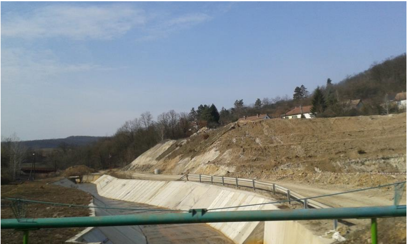
Figure 4 Waste from historic mining operations at Lahoca Hill to right of image. Channelized stream has largely eliminated direct erosion into the biosphere. Funded by Hungarian government.
