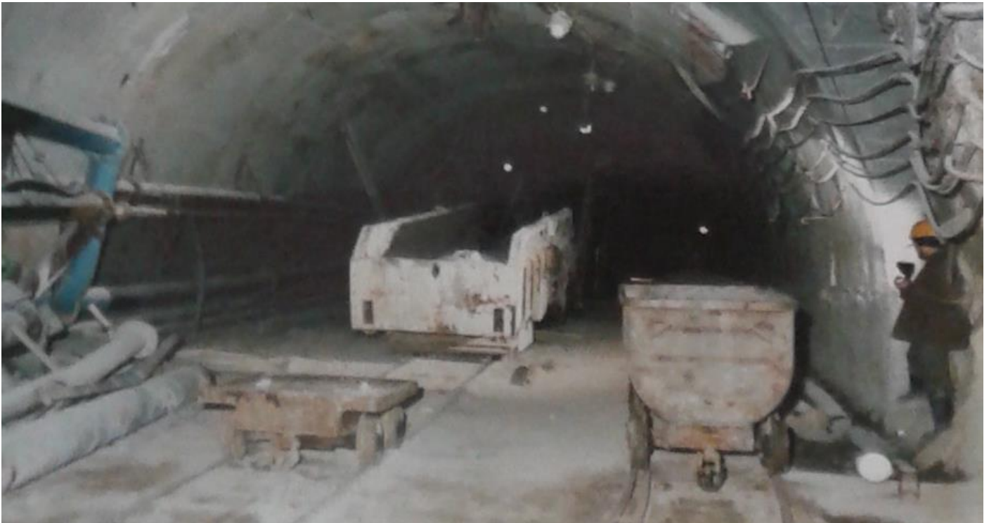
Figure 3 700 metre development level Recsk, Hungary. View from shaft along the main drive. (Photo undated, note level now flooded).
